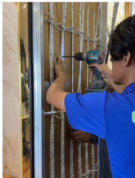
STEP 2 – LED Matrix Installation
