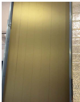
STEP 1 – Frame Preparation
