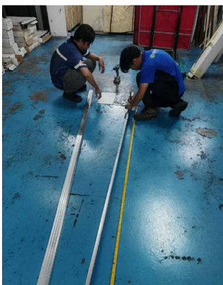
STEP 1 – Measure Wall & Plan Frame Size
